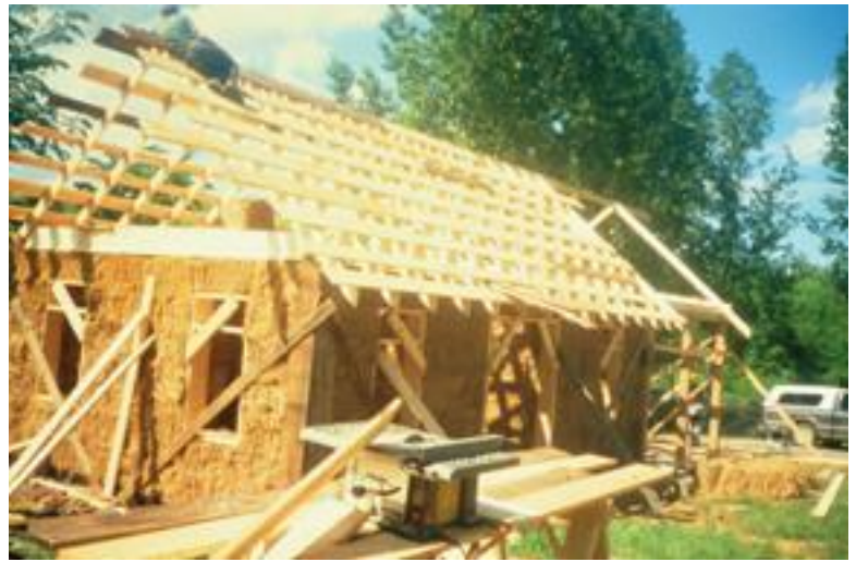
Building with straw bales.
